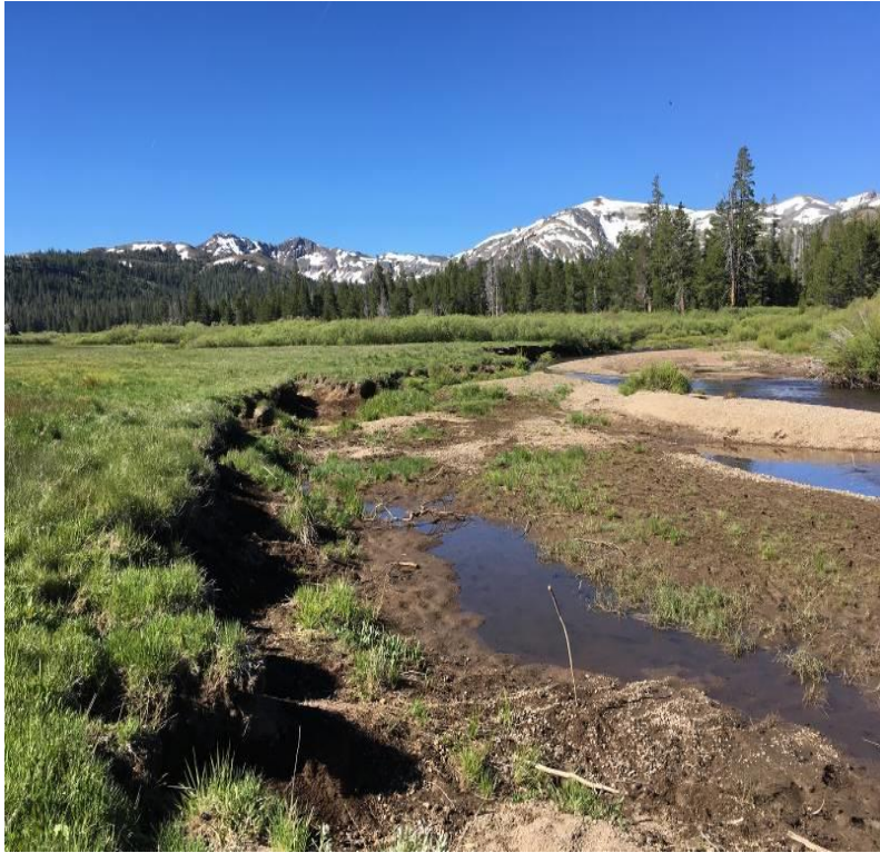
Figure 16. Saturated area within existing floodplain where willow and sod plantings could help anchor the streambank.
